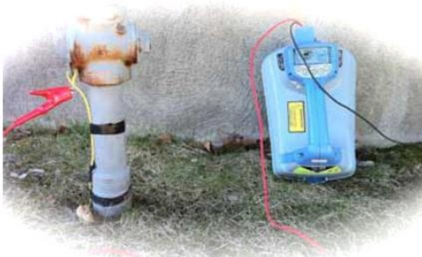
Direct connection to gas service tracer wire
