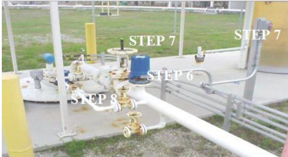
Cleaning OWS – Underground Process Tank
