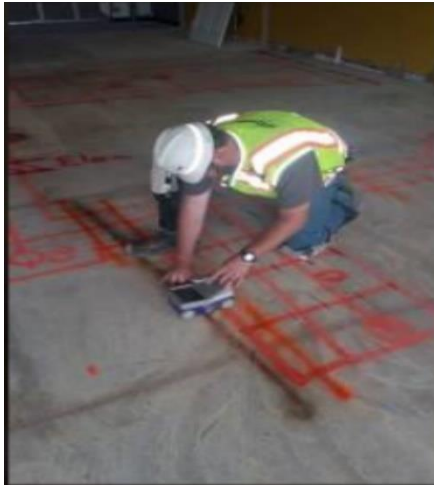
Figure: High Resolution Concrete Scanning (Source: Pennhaul Technologies)
