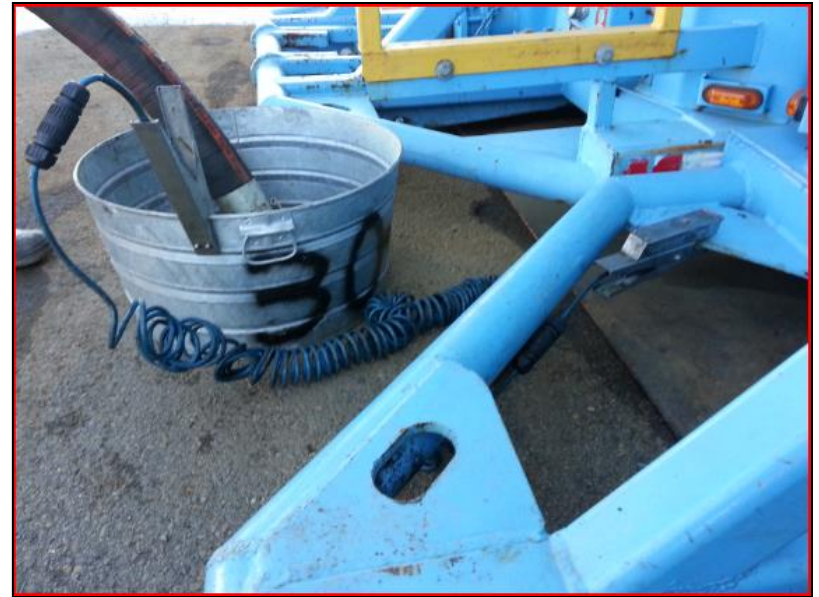
Bond of conductive container to a steel tank, (shown using indicating bonding cable that lights when bond is <10 ohms)
